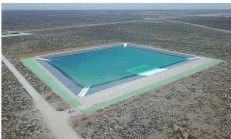
Liners & Pit Construction
