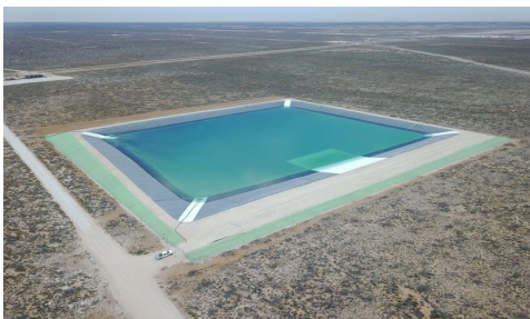
Liners & Pit Construction
